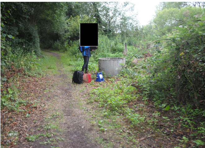
BH 704 on footpath to east of Nursery
