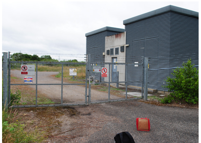
Secure compound containing BH 704
