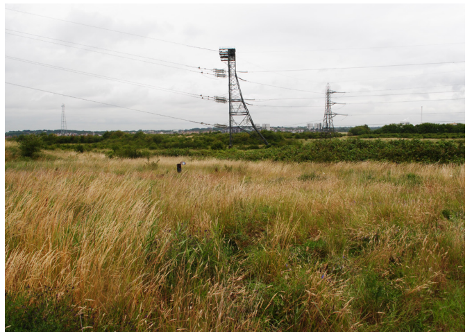
Old destroyed well near WS202
