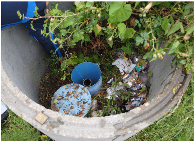
BH 707 – inside manhole ring
